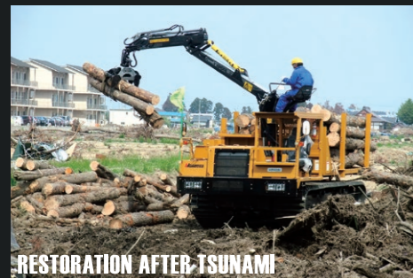
RESTORATION AFTER TSUNAMI
